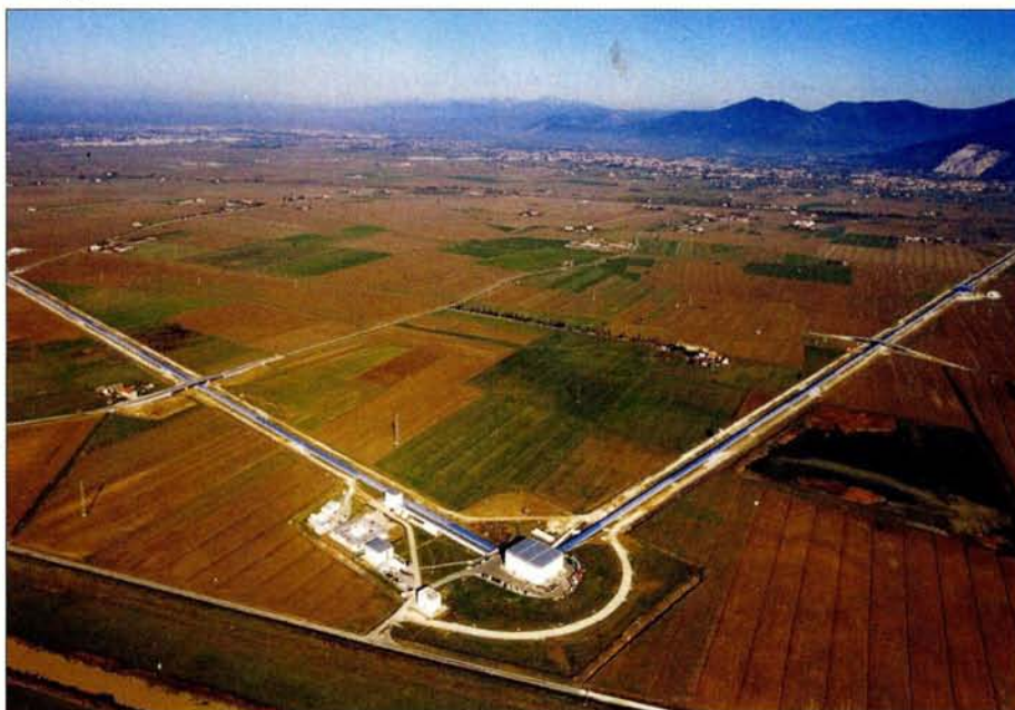
An aerial view of the Virgo site in Cascina, Italy. The Virgo Gravitational Wave Interferometric Detector is being commissioned and the participants visited it at the start of the meeting.
